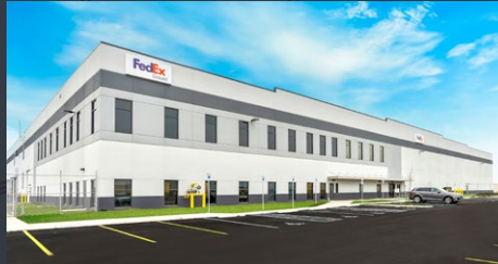
FEDEX GROUND DISTRIBUTION CENTER Bowling Green, OH | 250,956 SF Closed 4/5/2023
