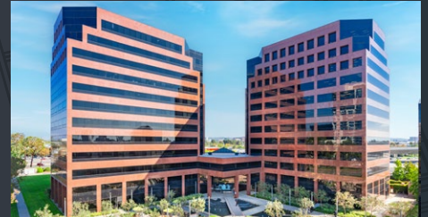
GRIFFIN TOWERS Santa Ana, CA | 560,163 SF Closed 4/6/2023
